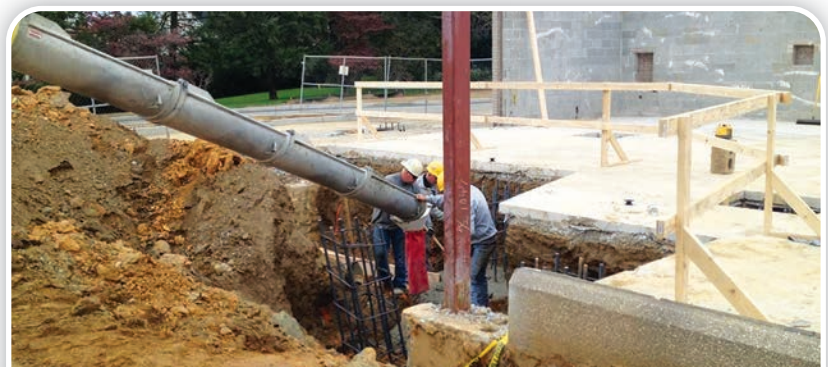
CONSTRUCTION AT THE FUTURE WEST CHESTER LOCATION
